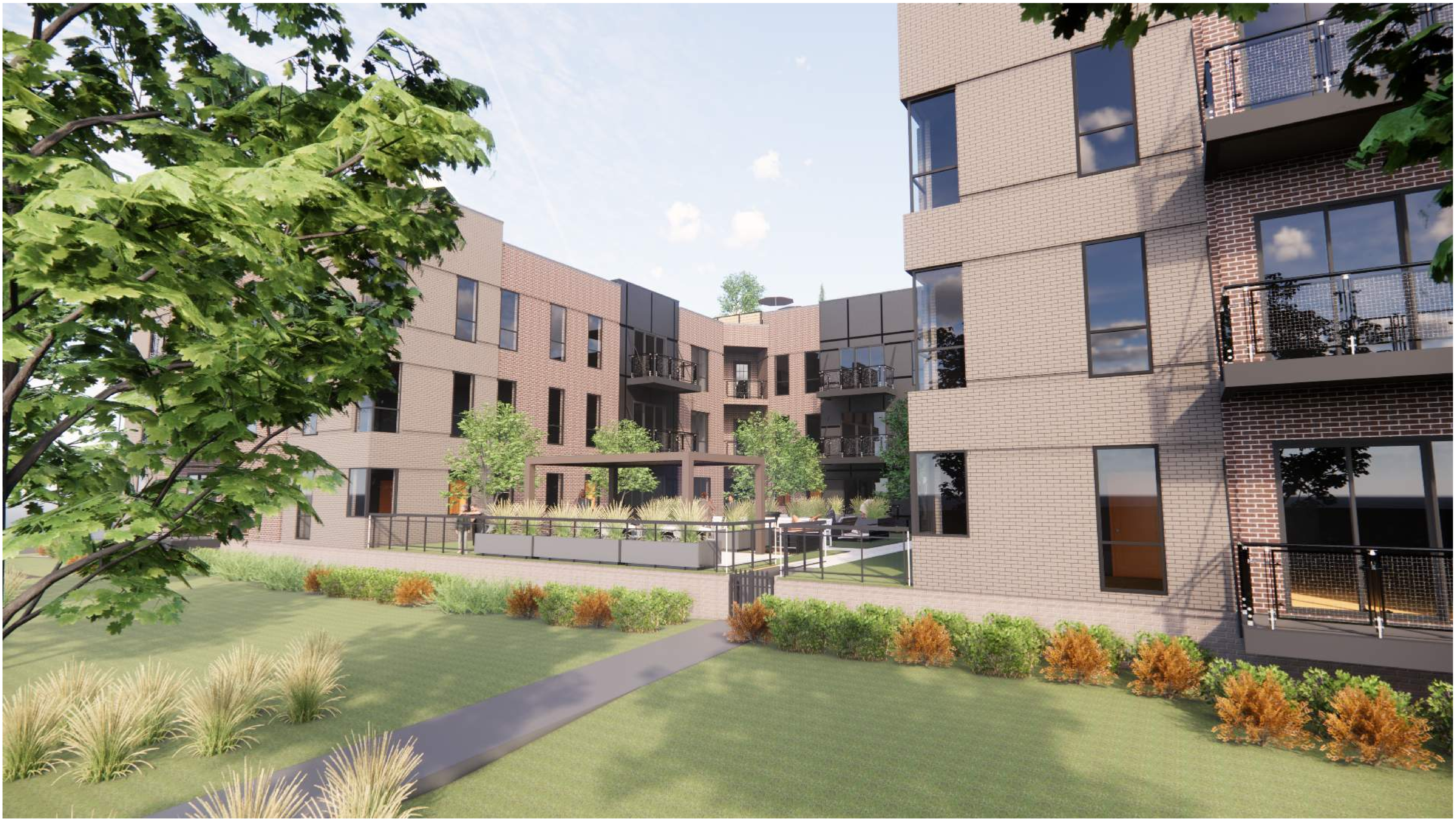
WEST - FACADE VIEW @ SECOND FLOOR TERRACE
