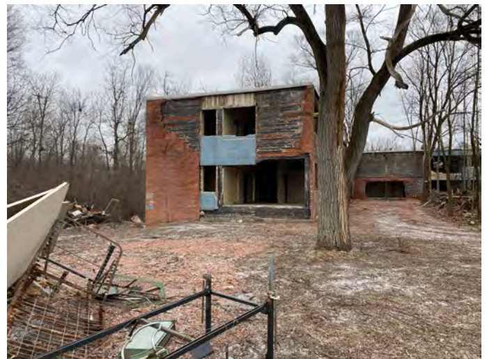
Former State Psychiatric Hospital; Exterior Building 11
