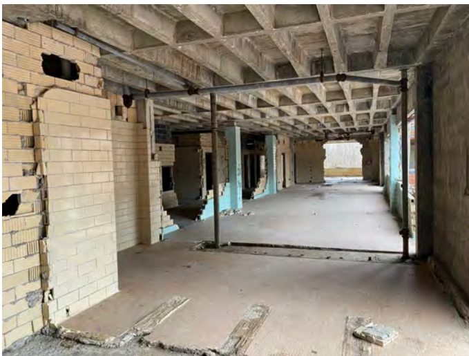
Former State Psychiatric Hospital; Interior Building 11
